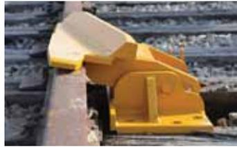
**Too Low.** A derail block that does not lie flat will cause a failure to derail.
