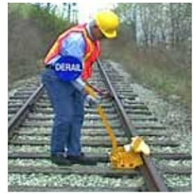
Always lower and raise the derail sign when you remove or reinstall the derail block.
