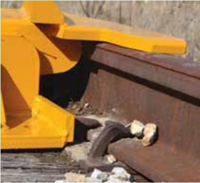
The derailer sits on two ties and must be pushed up against the rail head. The tie plates inside the rail will get in the way, so it is necessary to crop the plates close to the base of the rail. The derailer base must sit flat on the ties.
