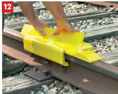
**12** Test tightness of derail on rail.
