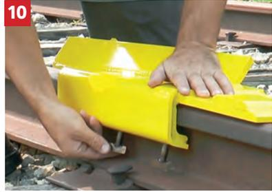
**10** Hand-tighten thumbscrews on field side.
