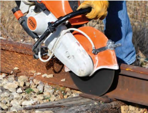
Mark each tie plate about an inch away from the rail base. Use a metal-cutting power saw or a torch. If using a saw, remove the spike on the gauge side and cut the plates. If using a torch, you will need to remove the two tie plates from under the rail, crop them, and then reinstall them under the rail, re-spike the outer portions of the plates.
