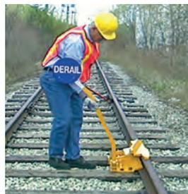
Always lower and raise the derail sign when you remove or reinstall the derail block.
