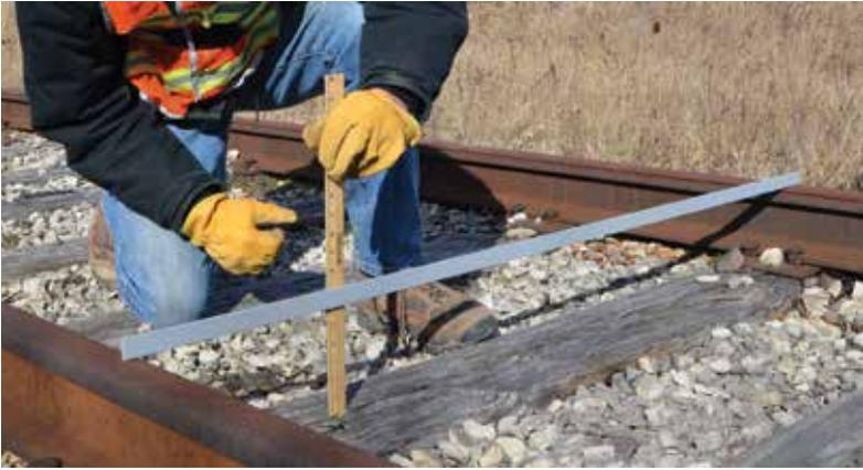
***To be effective, a derail must be correctly sized for the rail it is installed on, and adjusted in height so that the derail block (the part that swings onto the rail) lies flat on the surface of the rail.***
