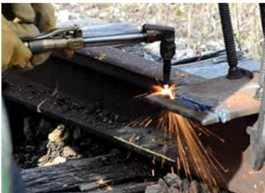
***Do not, as a short cut, permanently remove the tie plates. They are needed to support the rail and hold to gauge.***
